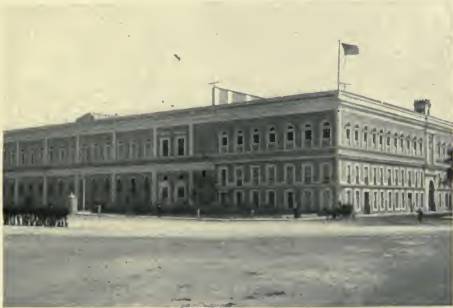
THE PRESENT POST-OFFICE BUILDING
